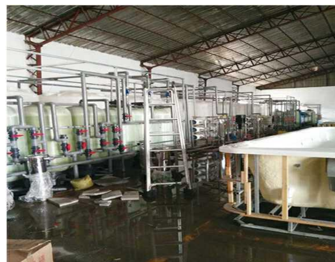
大型车用尿素安装现场 Installation site of large vehicle urea
